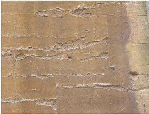
**Fig. 5.** Decay of a Jurassic oolitic limestone initiated along clay partings within the stone, Oxford (approximate image width 1 m).
