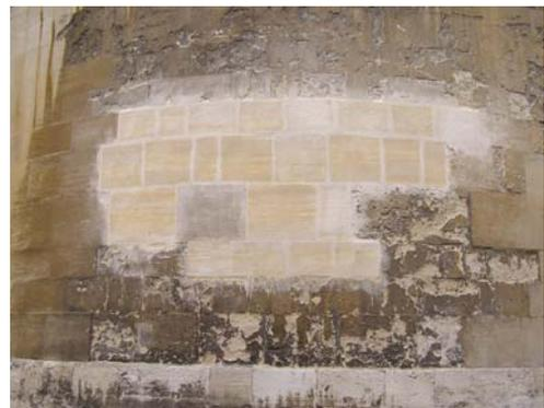
**Fig. 8.** Replacement of a section of wall in Oxford previously destroyed by catastrophic decay of Jurassic oolitic limestone (approximate image width 6 m).
