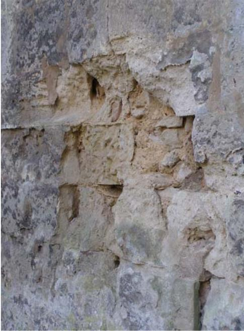
**Fig. 4.** Catastrophic decay of a section of wall constructed of Jurassic oolitic limestone, Oxford (approximate image width 4 m).
