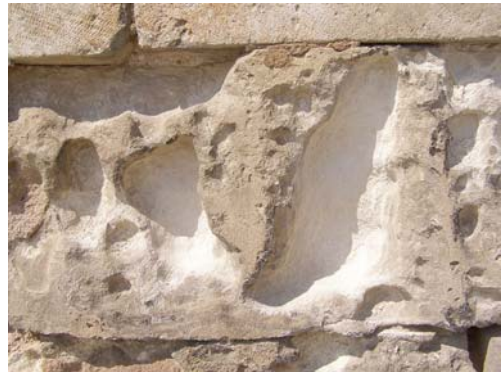
Fig. 2. Cavernous hollows developing on a Quaternary calcarenite, Mallorca (approximate image width 40 cm).
