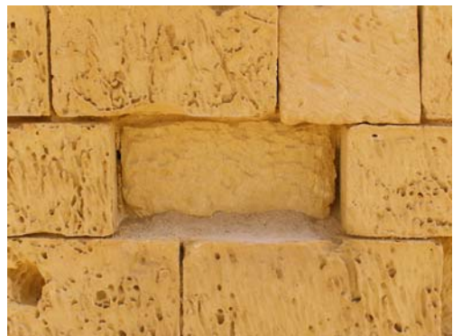
Fig. 3. Catastrophic decay of an individual block of Globigerina limestone, Malta (approximate image width 2 m).
